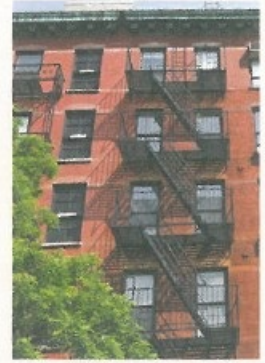
6 a fire escape
